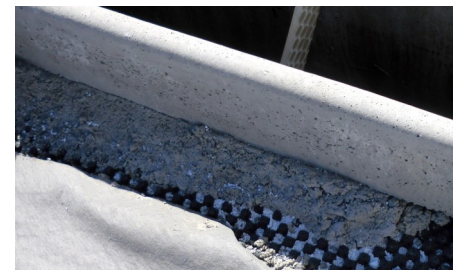
Floradrain® FD 25-E is used as permanent form-work for the separation between hard surface and garden.
